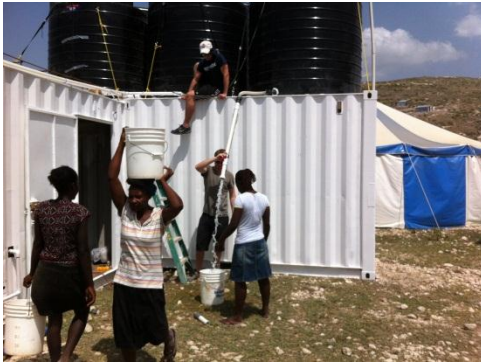
Figure 5: Three 1000 gallon tanks stored untreated and treated water. Two with clean, one with well water.
