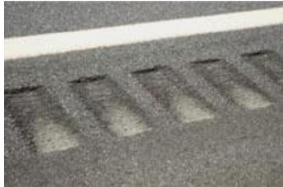
Figure 2.. Rumble Strip on a Roadway [Safe Roads 2003]
