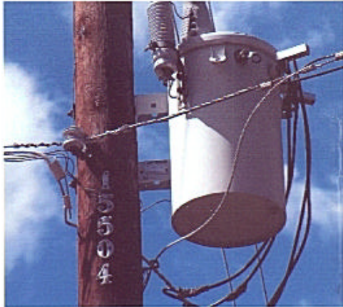
Figure 1. A 25-kVA Distribution Transformer
