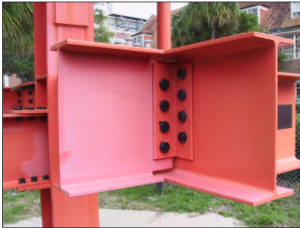
Fig. 3 Staggered, Bolted Double-Angle Connection on Steel Sculpture (View Looking northeast) Showing Beam Copes
