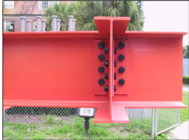
Fig. 4 Staggered, Bolted Double-Angle Connection on Steel Sculpture (View Looking East) Showing Double-Angle Framing
