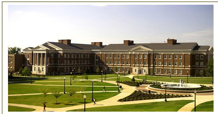
University of Alabama's Southern Engineering Research Center in the Shelby Engineering and Science Quad
